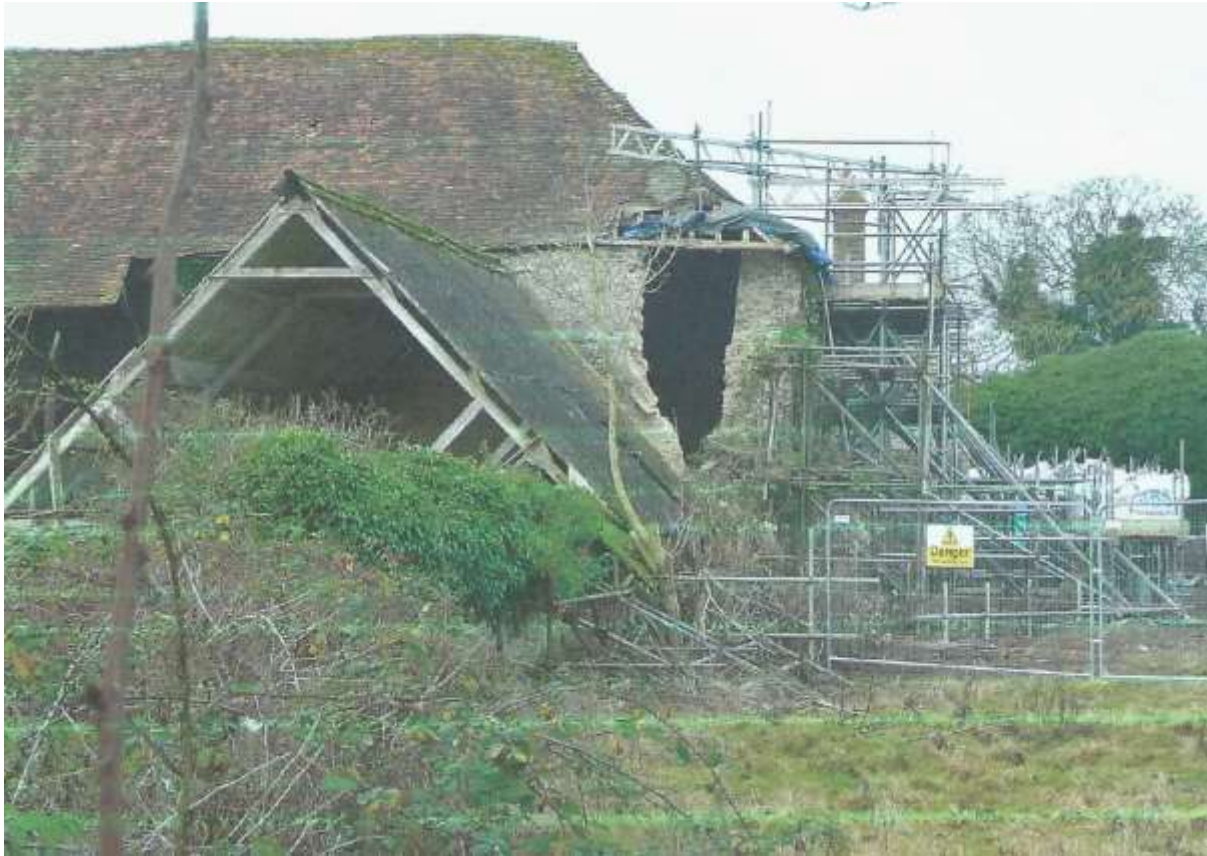
Figure 24: Charing Archbishop's Palace Great Hall, December 2016. The North-East corner has collapsed and the north wall leans out (Charing History Society).
